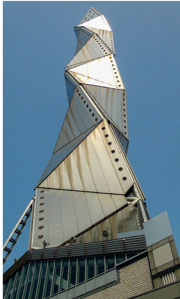
Figure 8.6 Art tower Mito in Mito, Ibaraki, Japan, by architect Arata Isozaki, is based on the tetrahelix. (Photo by CyberOyaki; CC by 3.0)
